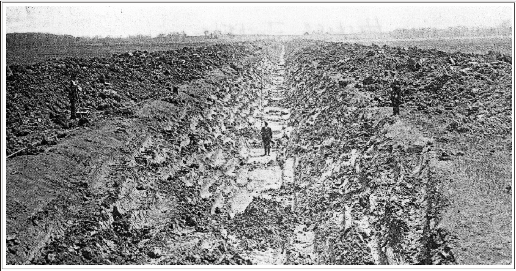
Figure 8. Central North-South Drainage Canal Under Construction in the Baker Wetlands, 1919.
